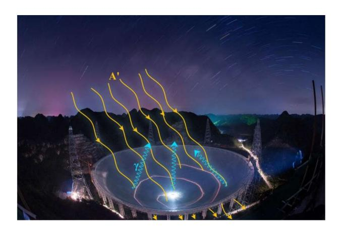
The dark photon dark matter has a small probability converts into visible radio wave at the dish of Five-hundred-meter Aperture Spherical radio Telescope (FAST), but may be detected at the feed of the telescope. Credit: Xinhua
